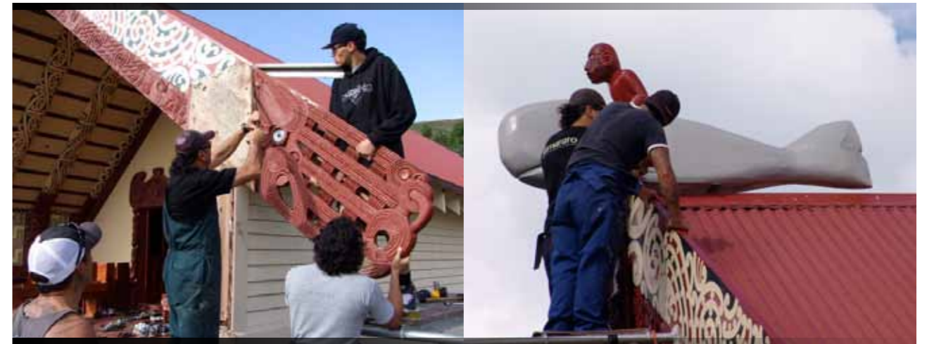
Whangara Marae Restoration Project
